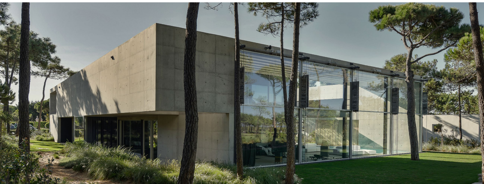
The Wall House, Portugal Guedes Cruz Arquitectos ©Ricardo Oliveira Alves
